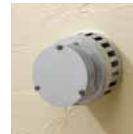
Balanced Flue (No chimney required)
